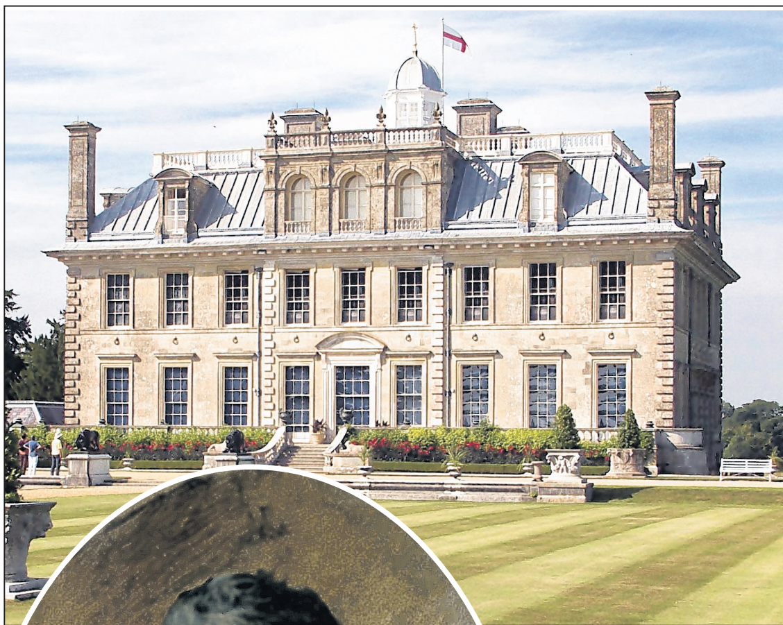
PIONEER: William John Bankes (1786-1855) by Sir George Hayter (1792-1871). Collector and traveller, rebuilt Kingston Lacy (above) to Sir Charles Barry's designs 1835-40. ©NTPL/Angelo Hornak
